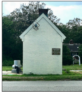
This is the existing 48th Street sewage pumping station today.
