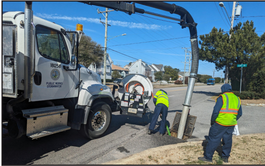
Working this truck in February to clear storm drains along Atlantic Avenue were longtime city employees Warren Powell and Gregory Sharp.
